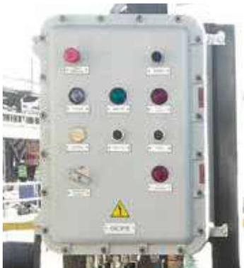
**A simple local control panel**, governs the hydraulic unit and possible accessories, such as acoustic and visual signals, movement restriction elements, removal cycles, operational limit detectors, instrumentation, etc.
